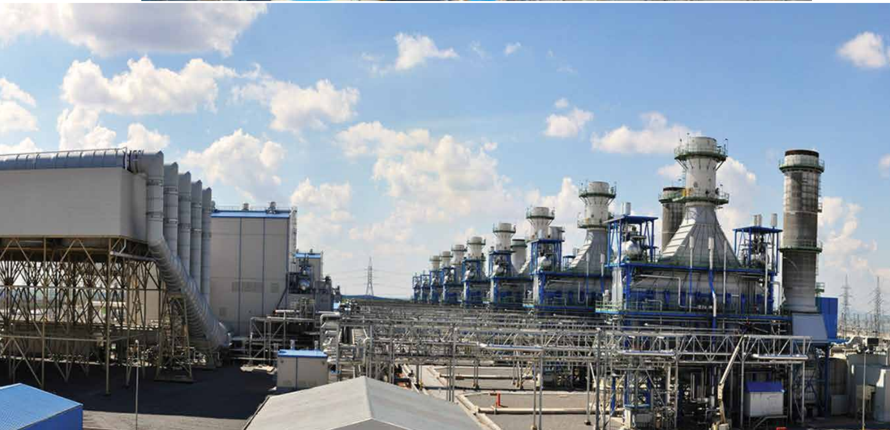
BESMAYA POWER PLANT
