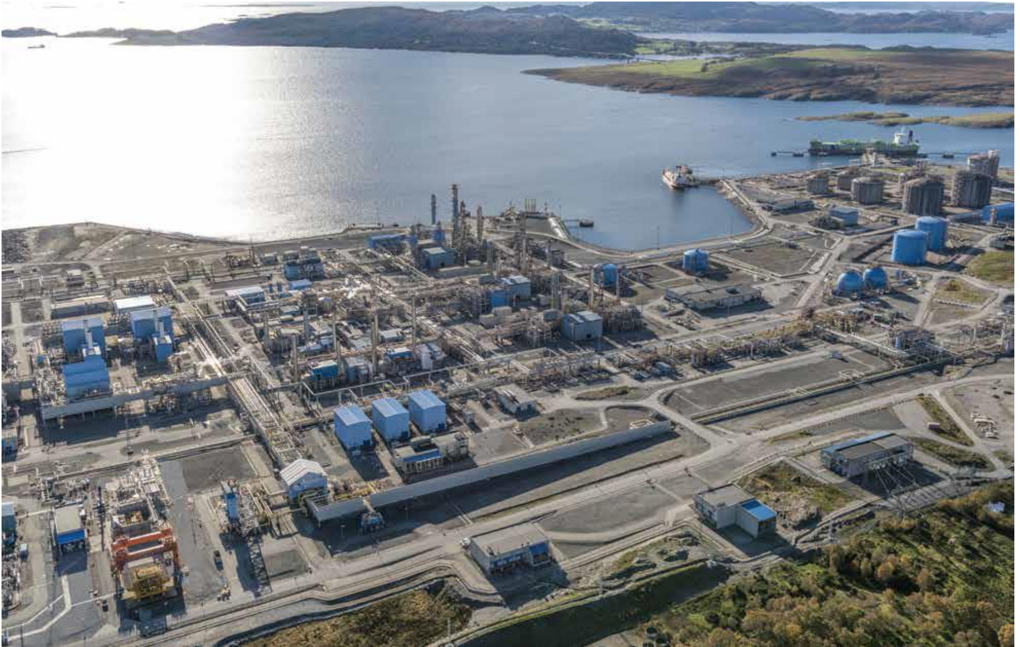
STATOIL KARSTO REFINERY
