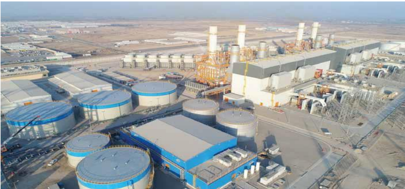
Besmaya Power Plant
