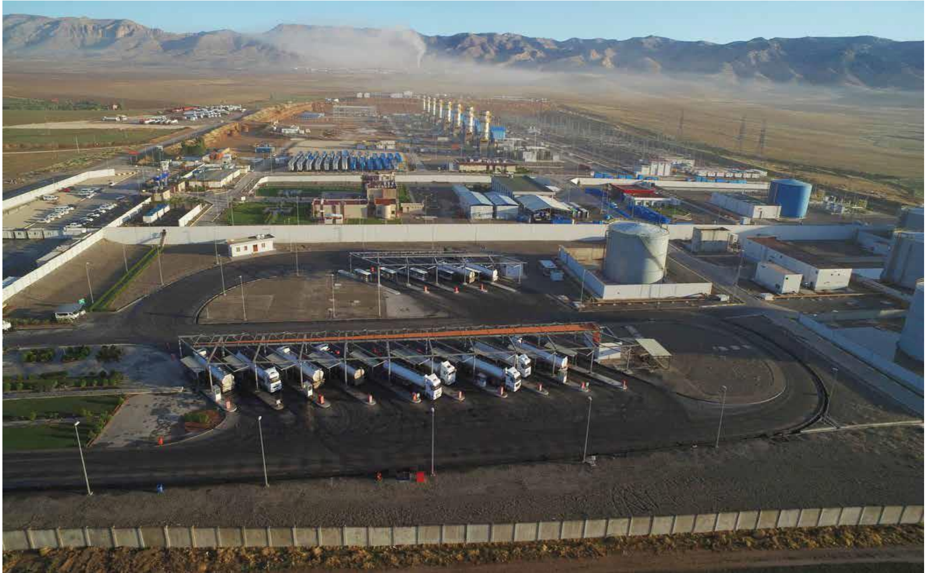
DUHOK POWER PLANT
